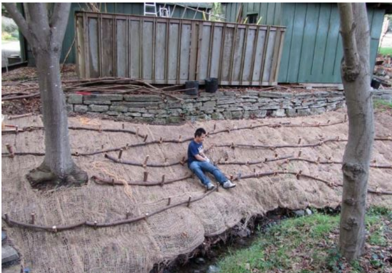
Figure 3. A student stakes down a geotextile fabric on the northern bank of the upper reach of Cerrito Creek within Blake Garden. Upper reach of Cerrito Creek Phase 1 restoration, February 2012 (Blake Garden).
