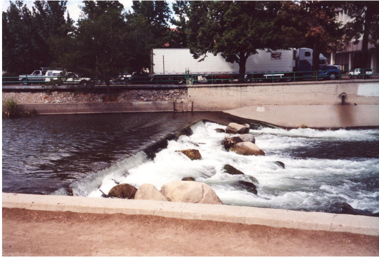
Figure 5: The Arlington Dam severely restricted fish passage and eliminated habitat heterogeneity in the North Channel at Wingfield Park. A similar diversion dam three miles upstream was measured in this study to replicate pre-project conditions in the North Channel. Photo sourced from Recreation Engineering and Planning.
