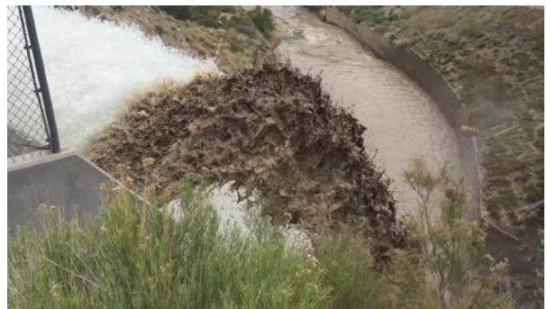
s. Sediment releases down the spillway of Millsite Dam near Ferron, UT (photograph courtesy of Rollin Hotchkiss).
