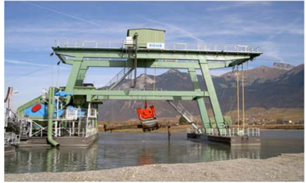
q. Mechanical dredging in Austria (photograph courtesy of Ellicott, Inc.).
