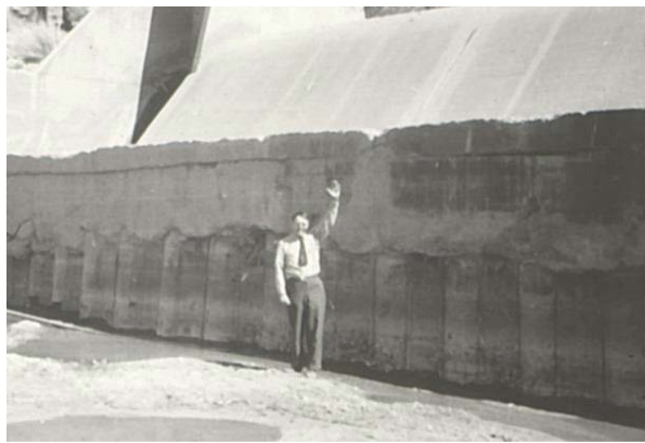
l. Channel degradation resulting from lack of upstream sediment source, downstream from Sumner Dam near Fort Sumner, NM.
