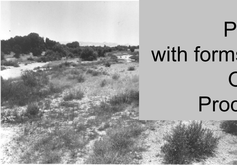
Figure 7.14 Uvas Creek channel viewed downstream from the Santa Teresa Rd bridge, the upstream end of the channel reconstruction project. (a) View in January 1996, shortly after November 1995 project construction. (b) View in July 1997, after the designed channel washed out in February 1996 and high flows in winter 1997 (from Kondolf et al. 2001, used by permission)
