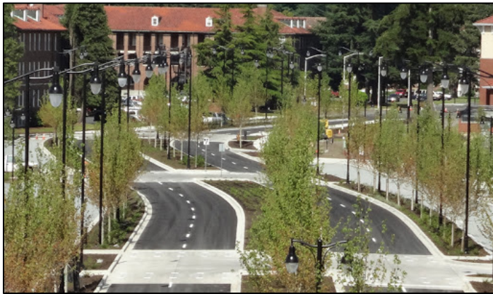
Figure 28. Pendleton Avenue on Joint Base Lewis-McChord, Washington, was redesigned with permeable paving and rain gardens, and now infiltrates 100% of runoff from the road. Source of image: 2019 Cascade Design Collaborative.
