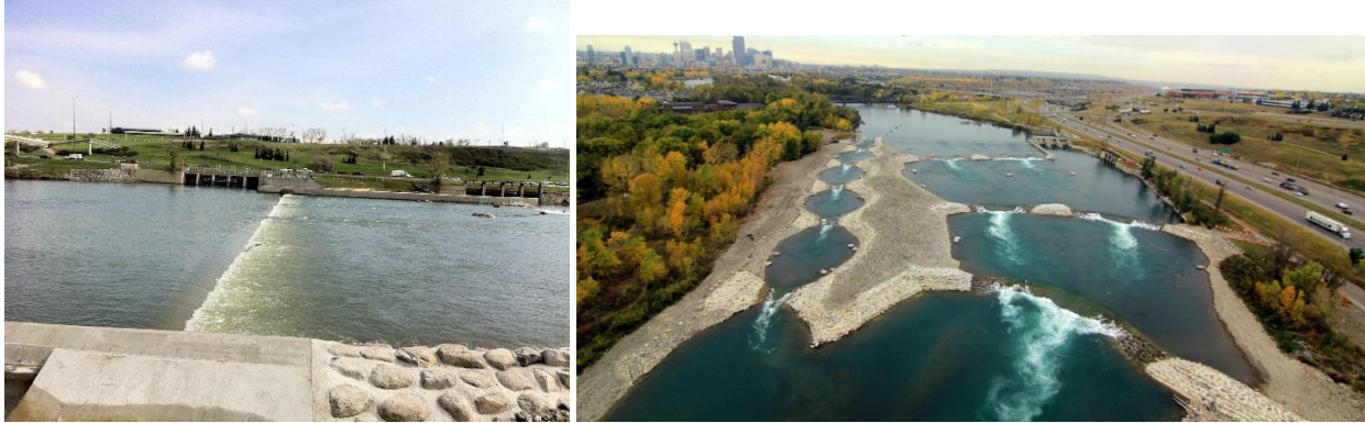
Figure 9: A low-head dam that drowned 11 people in Calgary, Alberta (left) transformed to a recreational amenity (right).
