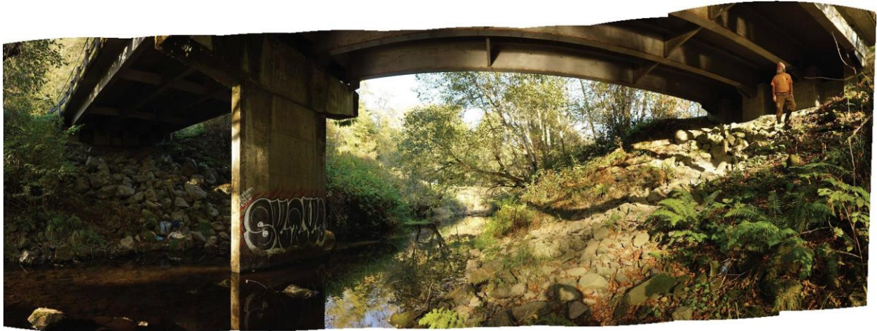
Figure 11. The narrowed Prairie Creek channel and confining structures of New Bald Hill Road overpass from both sides
