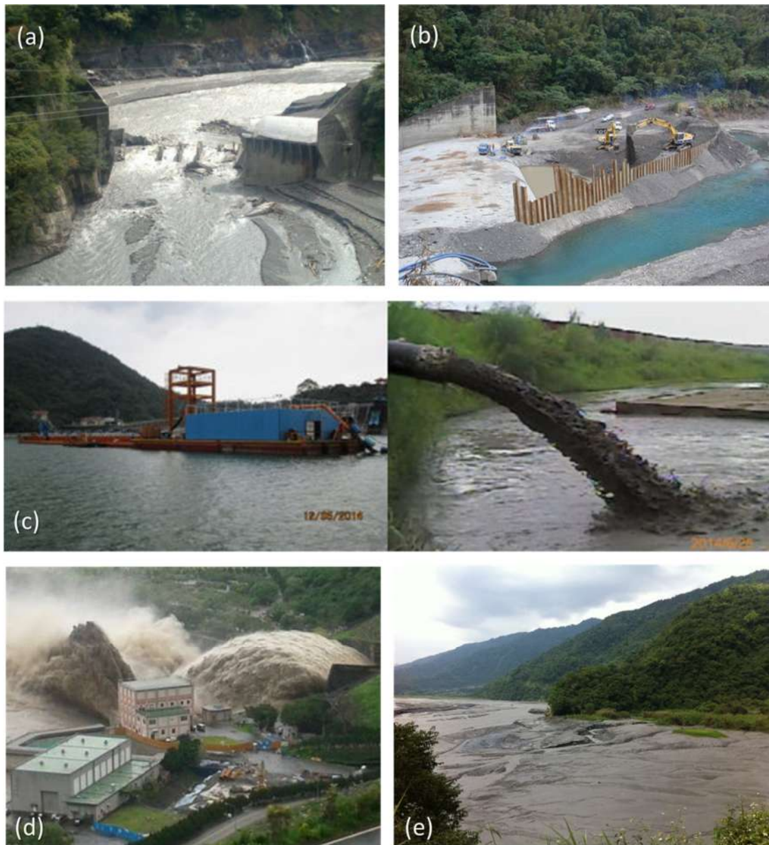
Figure 4. Images of sediment management strategies in Taiwan: (a) Barlin Dam, a failed sabo dam; (b) mechanical dredging from the lower most sabo dam, Yixing; (c) hydraulic dredging at Shihmen reservoir (WRA); (d) sluicing at Shihmen Reservoir during Typhoon Soulik in 2013 (WRA); (e) Drawdown flushing at Wujie Reservoir.
