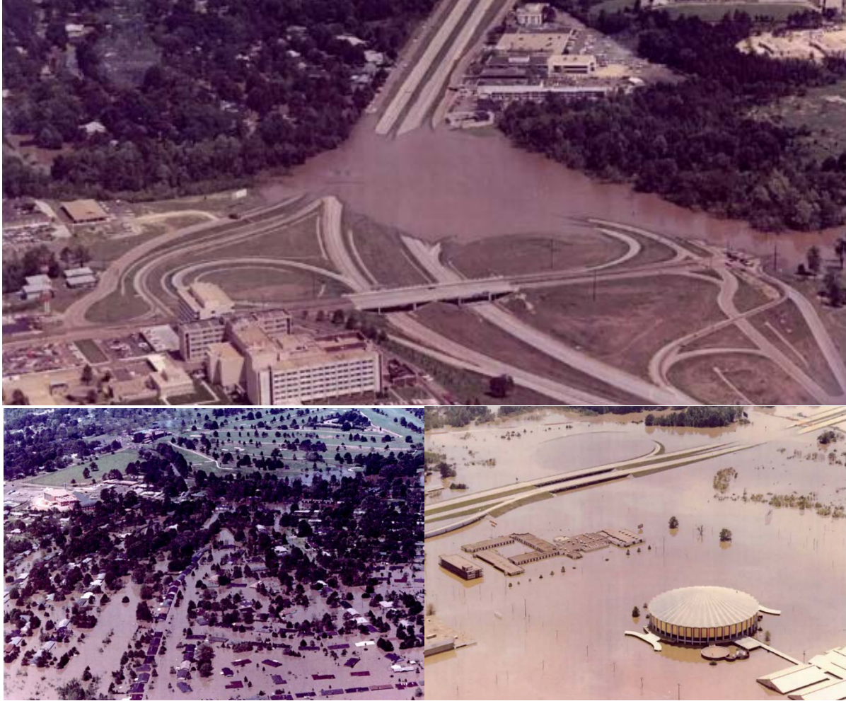
Figure 7: Flooding in Jackson, MS after the 1979 flood. Photos from The Clarion-Ledger.
