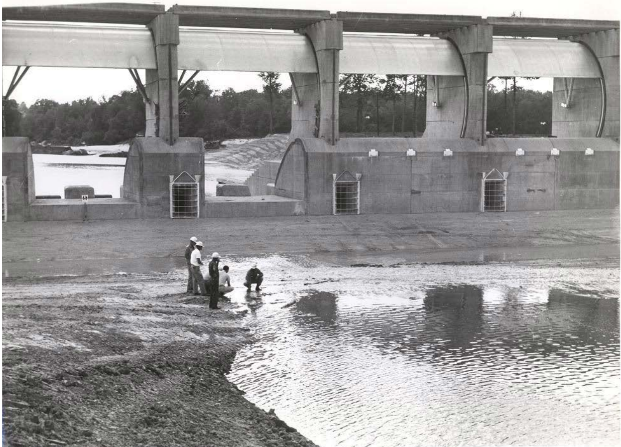
Figure 2. Construction of the Ross Barnett Reservoir Spillway in 1960 (Yancy, 2014).
